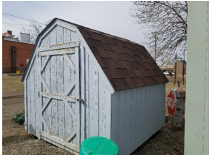
Figure 12 Storage Shed By Shop
