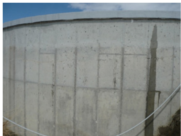
Figure 9 Concrete Water Tank
