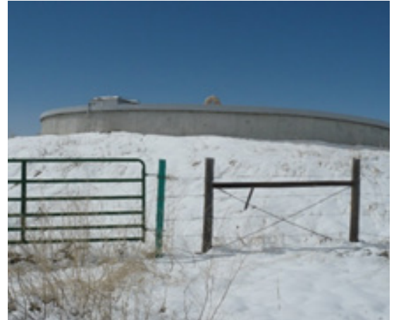
Figure 7 Concrete Water Tank
