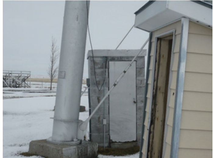
Figure 14 Tank SCADA Buildings
