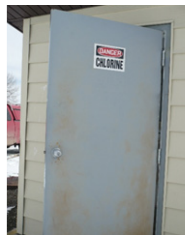
Figure 6 Disinfection Building Door
