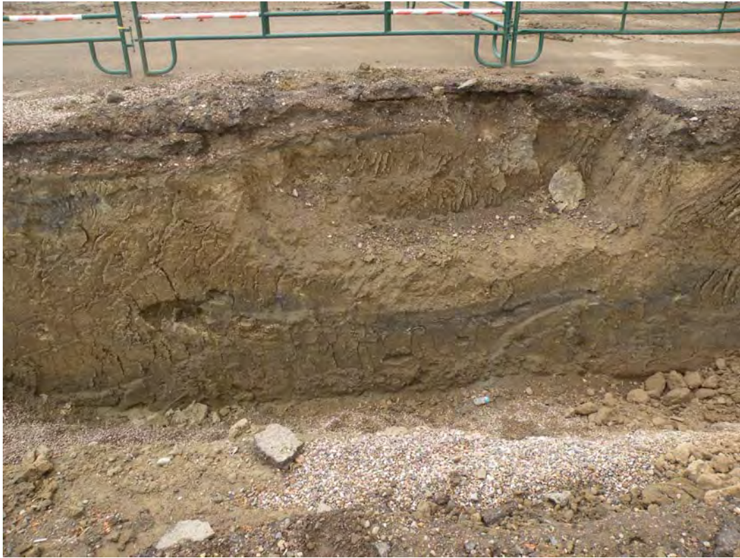
Trench wall – southern impacted area.
