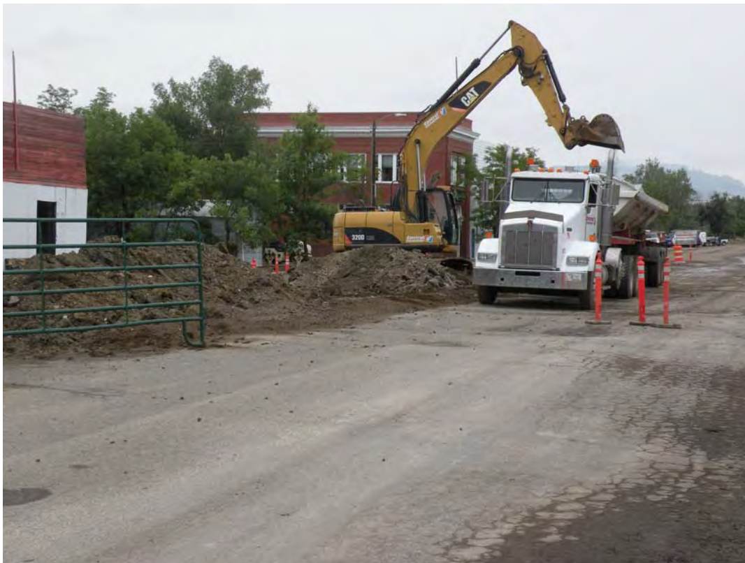
Loading Stockpiled Soil.
