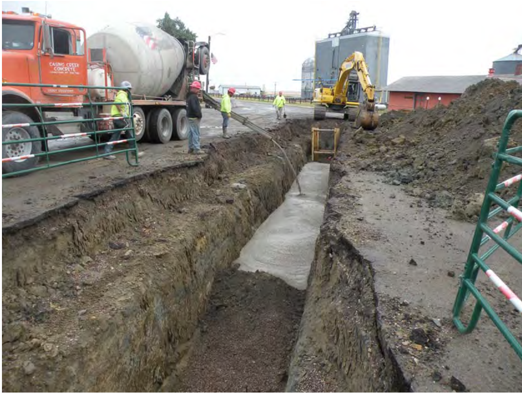
Emplacing flowable fill cap along north impacted area.
