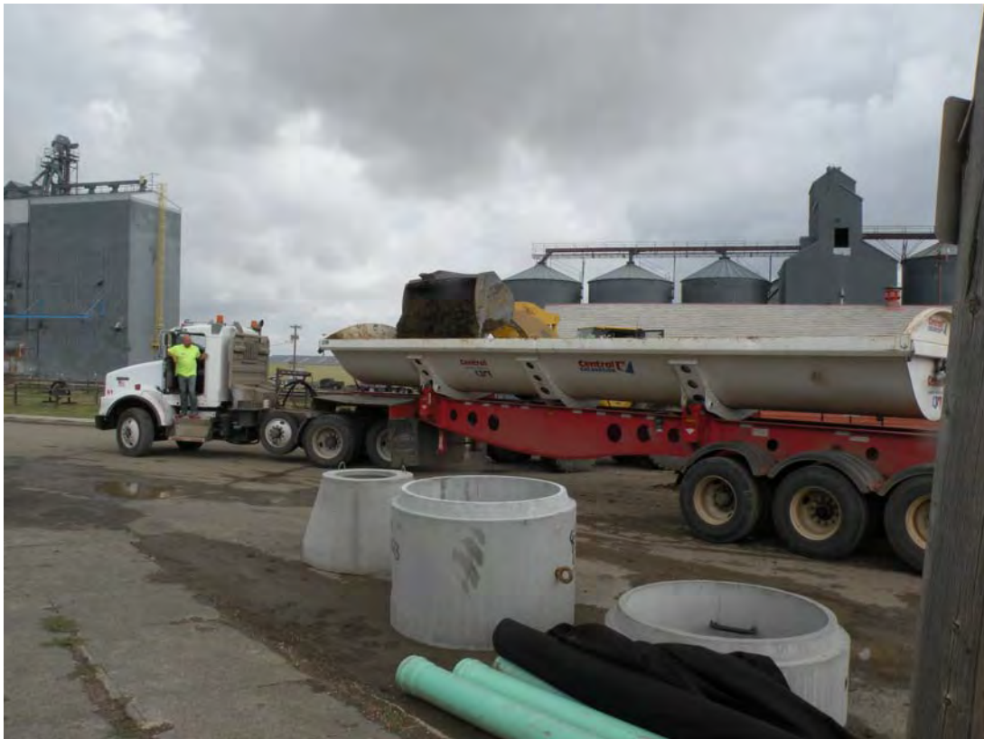
Loading soil from north impacted area.
