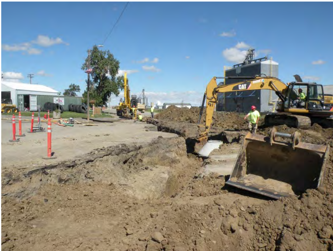
Trench looking north from end of impacted areas.
